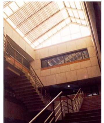
Roof integrated PV system
