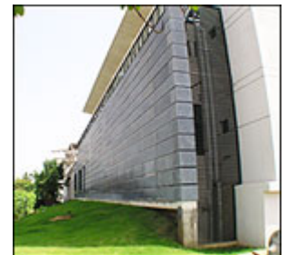
Solar wall cavity to aid ventilation
