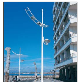
Suggested lighting fixture at Dwarka
