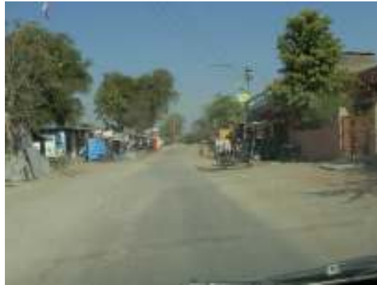
Bottleneck due to existing structure in village portion Sanwad
