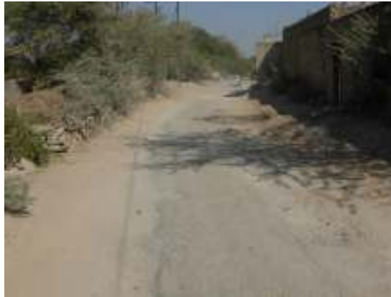
Bottleneck due to existing structure in village portion Anjana
